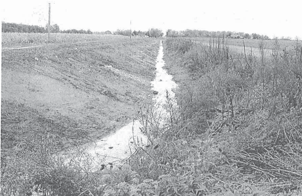
Figure 3: the 3-m deep municipal drain.
