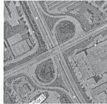
Figure 1: Sky view of the two exit ramps
