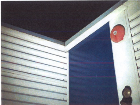
Figure 2.4 L2 northwest roof/wall corner
