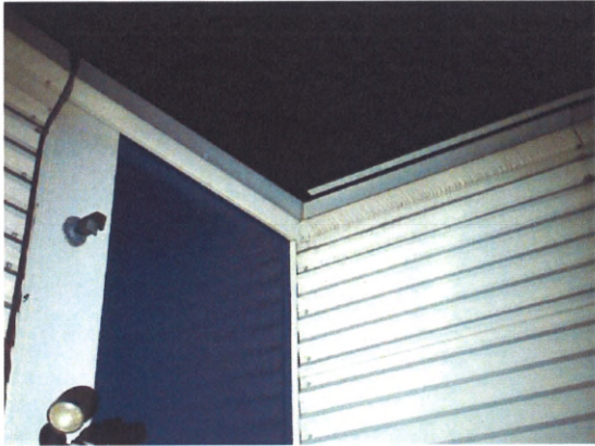
Figure 2.22 L2 southwest roof/wall corner
