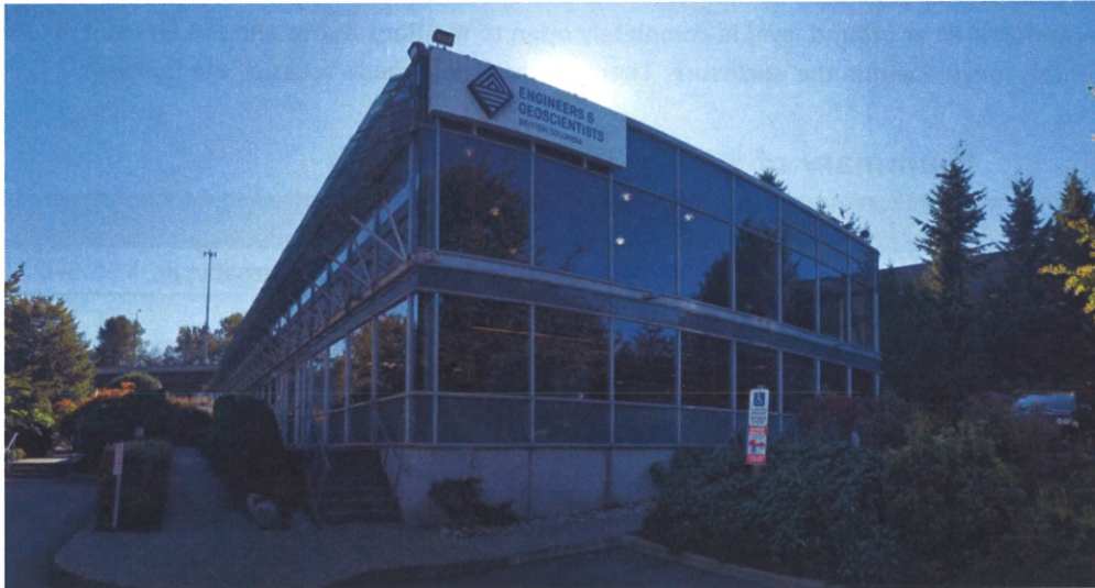
Figure 1: Photo (Northeast corner) of the Engineers and Geoscientists of BC office building.
