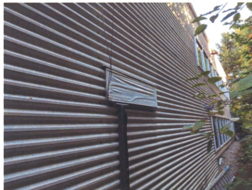
Figure 2 Exterior vents located on the West elevation were sealed using tape.
