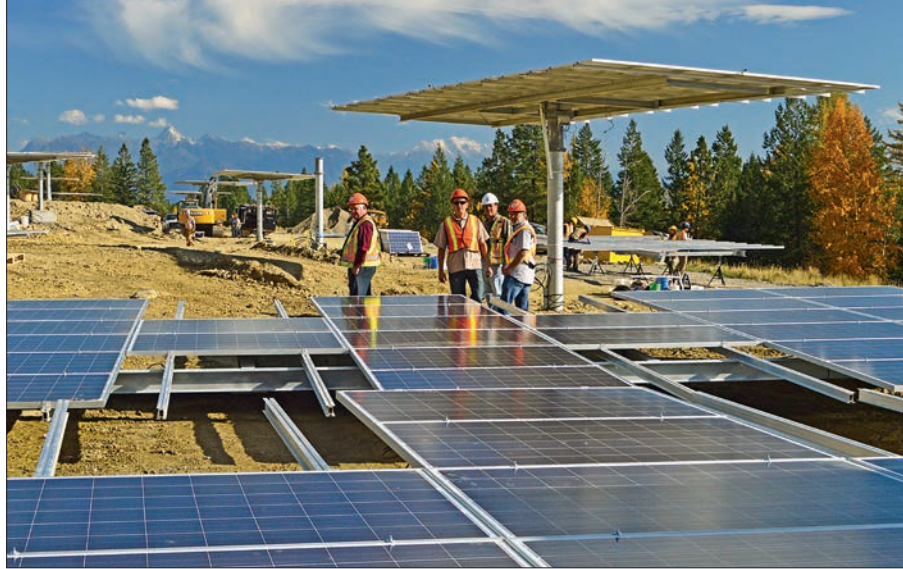
SunMine's solar panels are configured to allow up to 21 panels to be strung together, generating up to 1,000 volts instead of the usual 600 volts, and using less copper wire and electrical equipment. Photo: City of Kimberley
