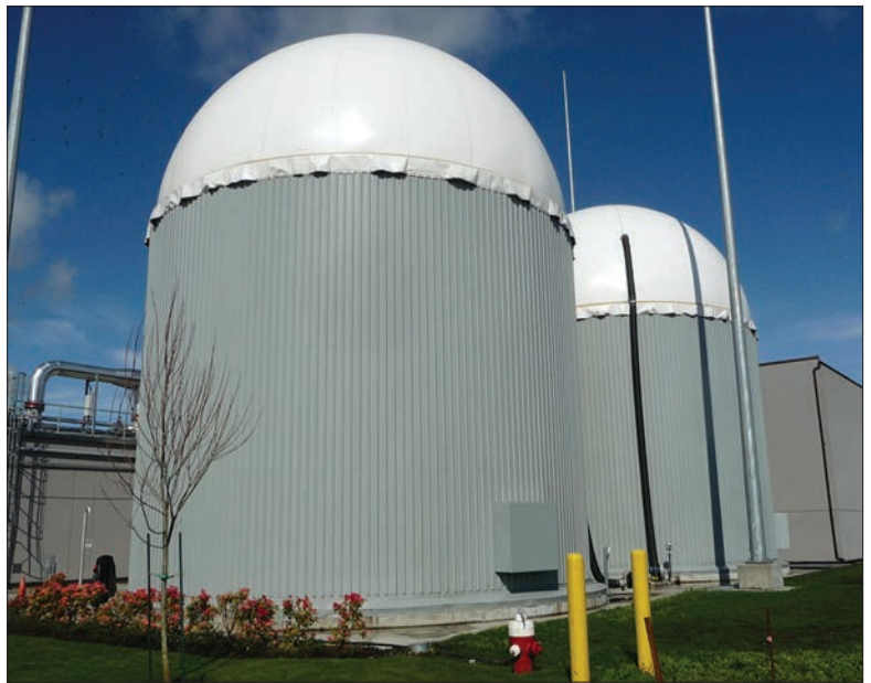
Harvest Energy Garden mimics organic decomposition in landfills. The percolator where waste is hydrolyzed and acidified, and the soluble organics are recirculated (recirculation pump system, left), the buffer tanks and digester tank (right) provide environments where anaerobic microbes break down the waste and release methane.
