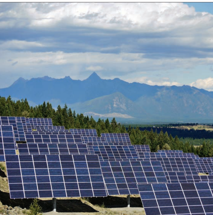
Kimberley, BC, typically sees a lot of sun throughout the year, with average solar energy yields for the area reaching up to 2,400 kWh/kWp per year. Those sunny skies provided opportunity to transform the decommissioned Sullivan Mine site into a 1.05-MW solar plant. Map: 2-Axis Mounting. Contour Map © EcoSmart 2014. Photos: City of Kimberley
