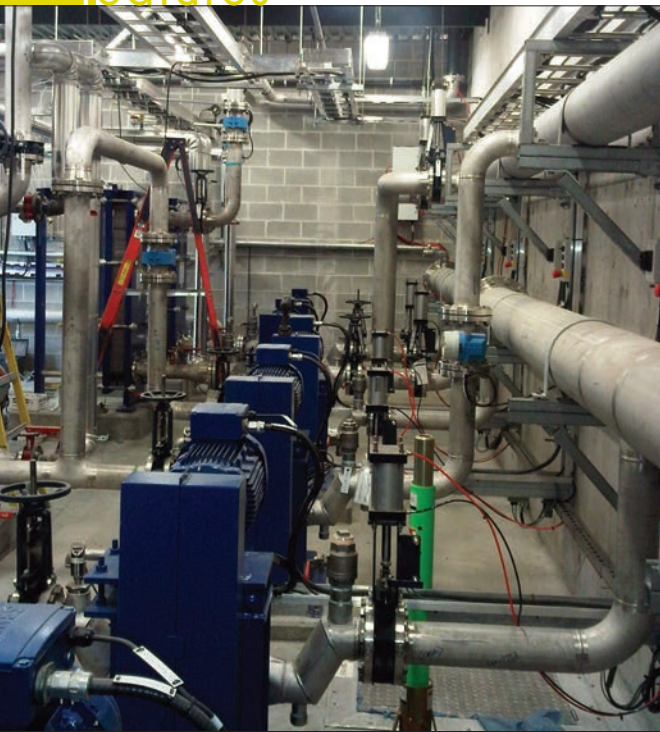
Harvest Energy Garden mimics organic decomposition in landfills. The percolator where waste is hydrolyzed and acidified, and the soluble organics are recirculated (recirculation pump system, left), the buffer tanks and digester tank (right) provide environments where anaerobic microbes break down the waste and release methane.
