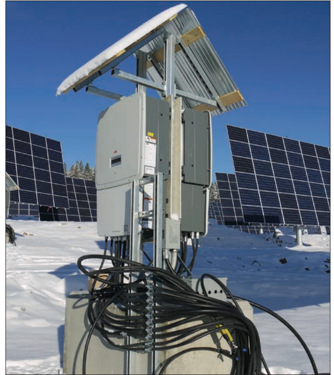
A dual-axis tracking system (left) that adjusts each panel's position to face the greatest amount of sun throughout the day generates up to 38% more solar energy than fixed-panel systems, and small DC-to-AC converters located close to the panels (below) cost less than using one central converter, are easier to maintain, and increase system flexibility, resilience and efficiency. Photos: City of Kimberley
