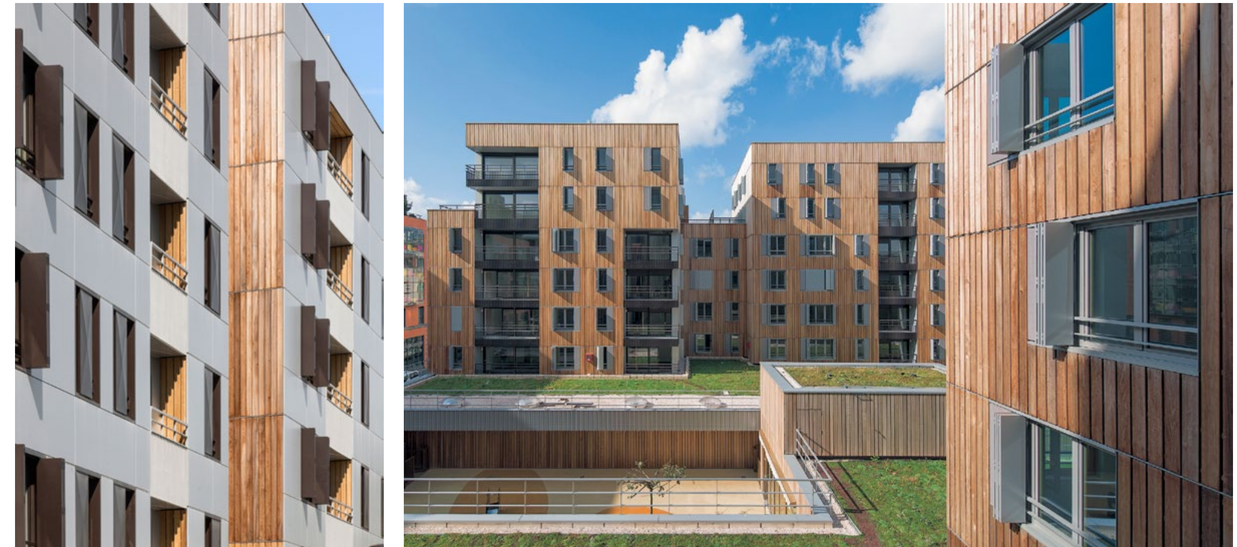
This mixed-use housing complex in Paris by Nunc Architects (2015) has varied façades some with exterior shutters that can be opened and closed to suit resident needs and climatic conditions. The architects aimed for double or triple orientations for each of the 107 dwellings on the site, and the design of articulated facades with shallow floorplates designed around daylight has created well-lit interiors. Photos Luc Boegly courtesy Nunc.
