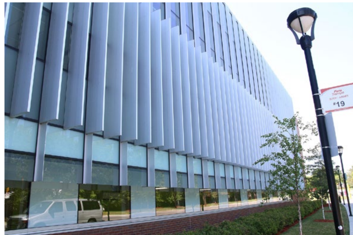
Example of side fins to protect occupants from direct solar radiation on an east-facing facade.
