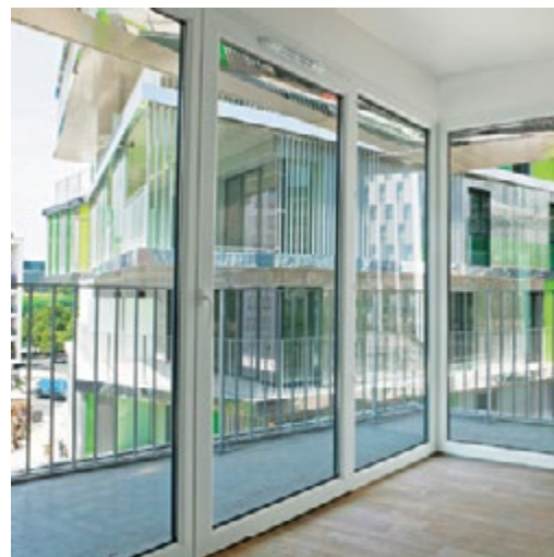
Very high window-to-wall ratios as shown on the left impact quality of life as residents sacrifice privacy, thermal comfort, and practicality. The photograph on the right shows housing with a lower WWR that still allows daylight, views, and connection to outdoors. (Right) Architects: LAN Residential Complex in Begles, France 2010.
