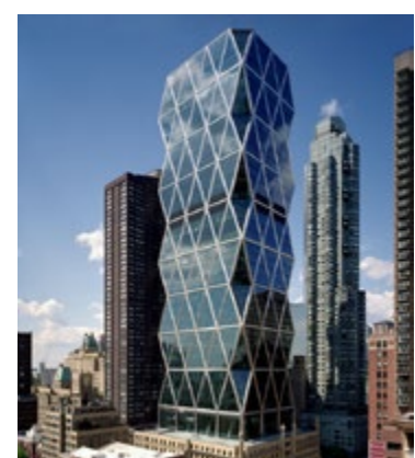
EXAMPLE: HEARST HEADQUARTERS, (2006) LOCATION: NEW YORK, NY, USA ARCHITECT: FOSTER + PARTERS DETAILS: THE DIAGRID SUPPORT STRUCTURE ENABLES A 20% SAVING OF STEEL. THE TOWER WAS BUILT TO 85% OF RECYCLED STEEL.
