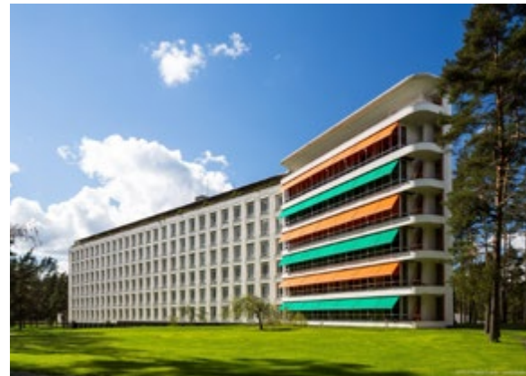
EXAMPLE: PAIMIO SANATORIUM (1933) LOCATION: PAIMIO, FINLAND ARCHITECT: ALVAR AALTO DETAILS: FEATURES SHALLOW FLOOR PLATES AND SINGLE-LOADED CORRIDORS TO MAXIMIZE DAYLIGHT PENETRATION AND CROSS VENTILATION
