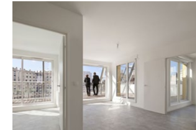
EXAMPLE: PLEIN SOLEIL (2013) LOCATION: PARIS, FRANCE. ARCHITECT: RH+ ARCHITECTURE. DETAILS: THE SOUTH FAÇADE FEATURES LOGGIAS WHERE EXTERIOR SLIDING PANES, PRINTED FOR THE BEDROOM AND TRANSPARENT FOR THE LIVING ROOMS, HELP MODERATE VIEWS AND CLIMATE ACTING AS SHADING IN THE SUMMER AND A THERMAL BUFFER SPACE IN THE WINTER. PHOTO: LUC BOEGLY.
