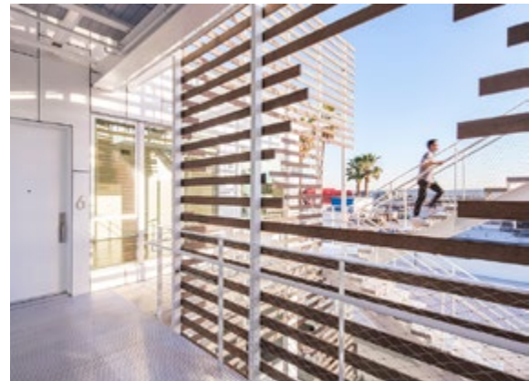
EXAMPLE: SAN VINCENTE 935 (2018) LOCATION: LOS ANGELES, USA. ARCHITECT: LORCAN O'HERLIHY ARCHITECTS DETAILS: THE EXTERIOR CIRCULATION PROVIDES WELCOME SHADING TO UNITS AND WALKWAYS. PHOTO © PAUL VU, COURTESY LORCAN O'HERLIHY ARCHITECTS [LOHA]
