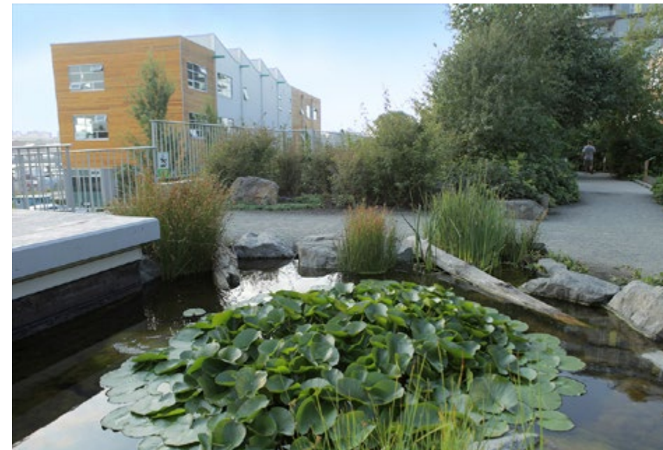
Dockside Green, a complex of multi-unit residential buildings and small-scale commercial buildings in British Columbia uses rainwater retention ponds and on-site sewage treatment to manage and conserve its water needs.
